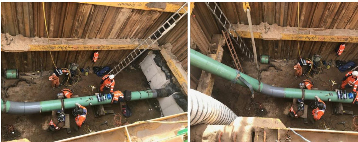
Figure 40 - Example of a Sheet Piled Excavation
