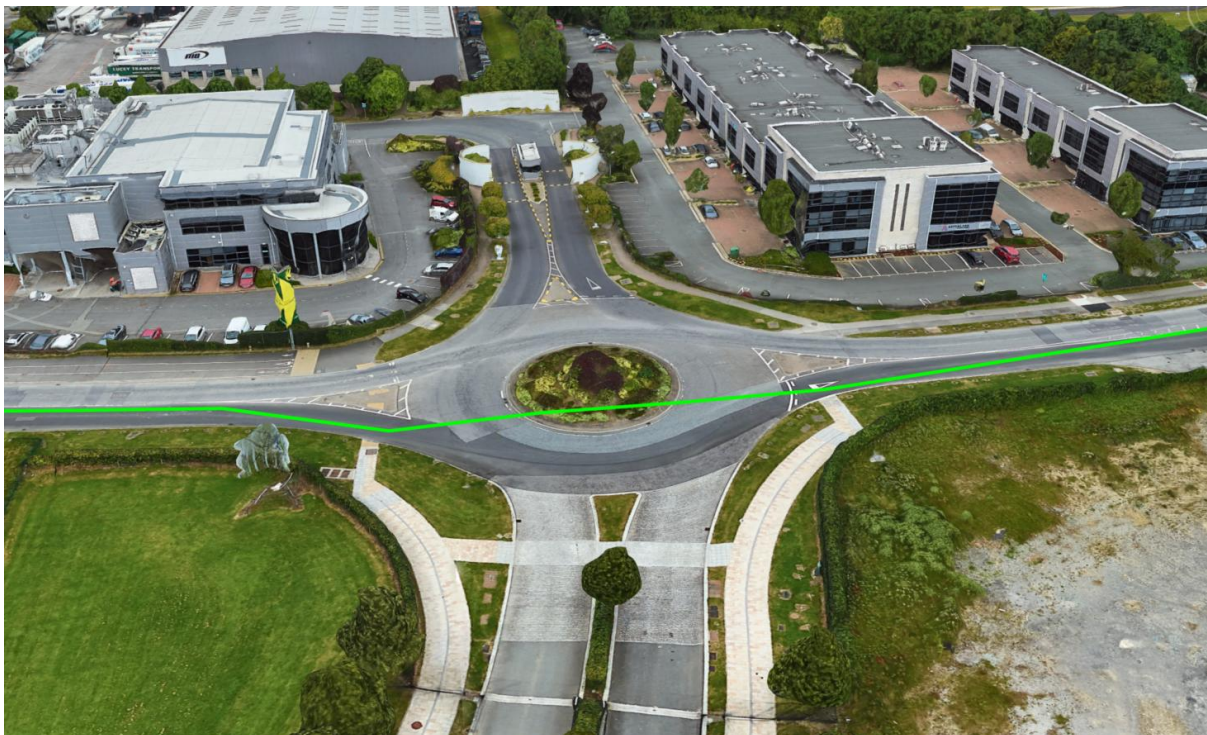
Figure 12 – Profile Park Roundabout
