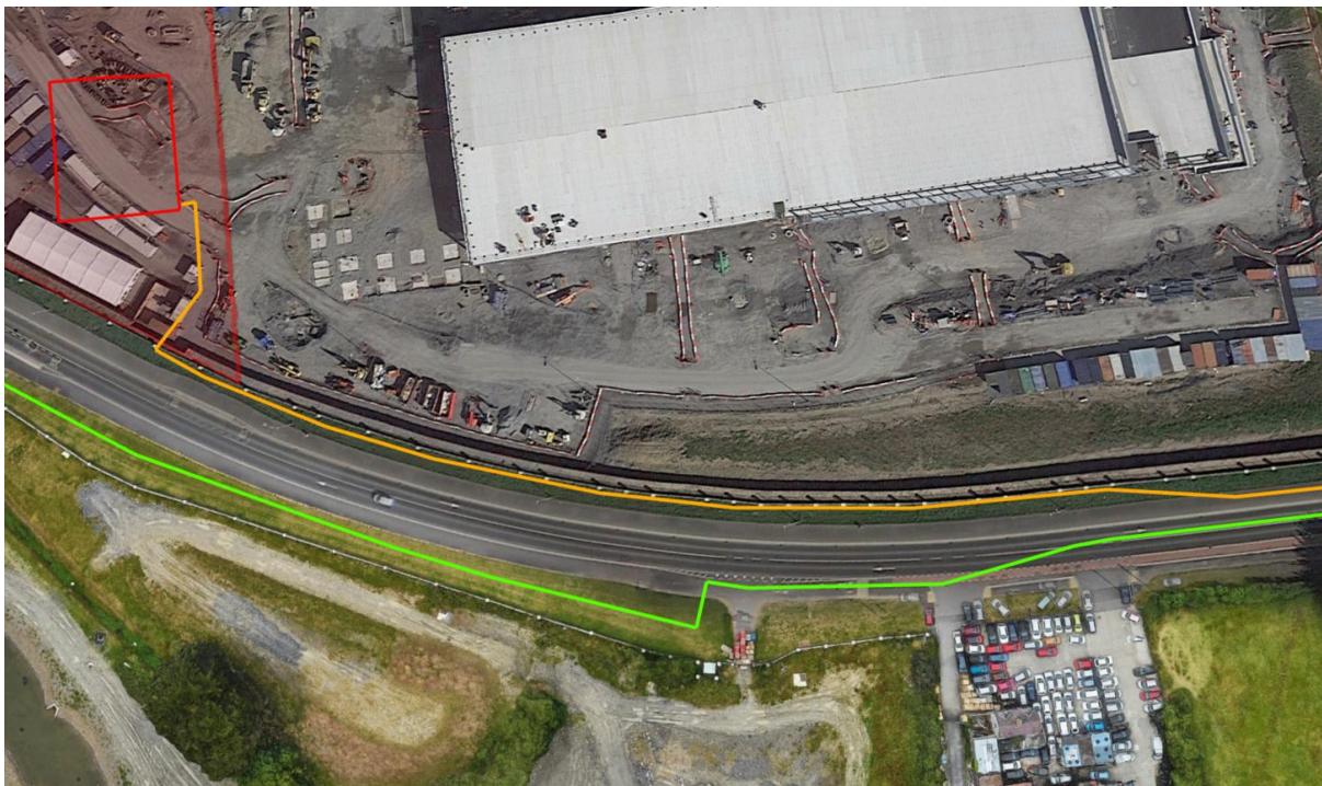
Figure 21 – GNI134 and GNI136 pipelines separate as two high voltage cables enter and run parallel along the R134 roadway
