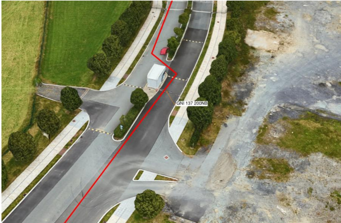
Figure 31 - Pipeline routing from the Nangor Road roundabout in the Profile Park Road
