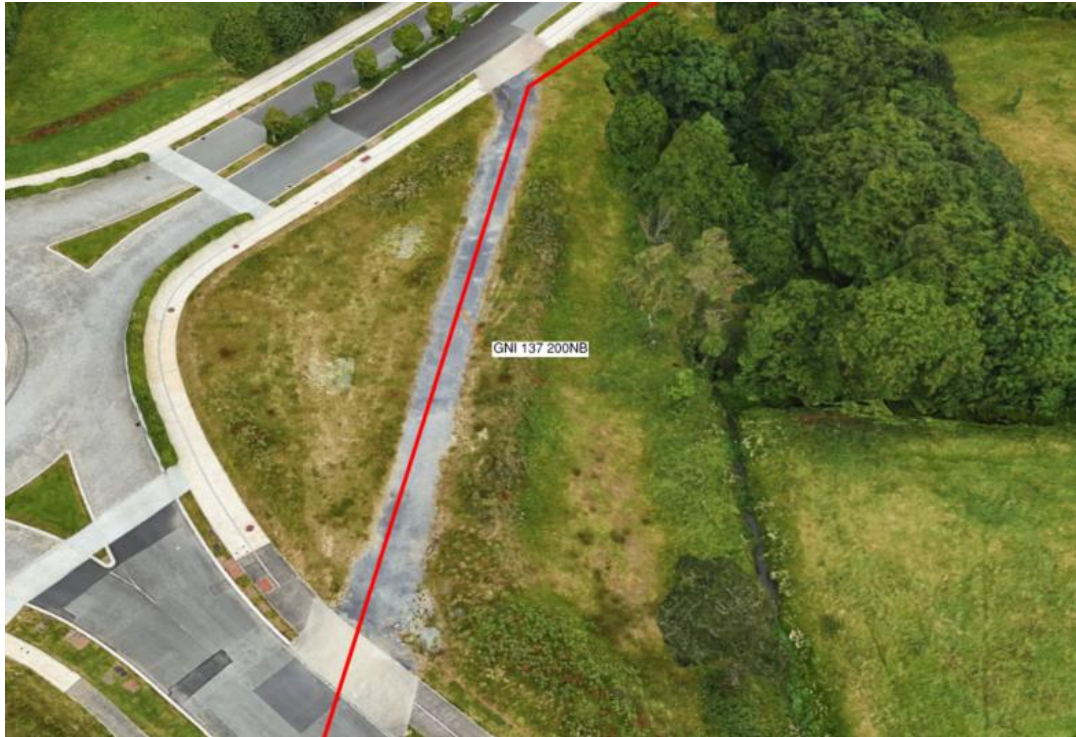
Figure 33 - Pipeline routing through the pathway adjacent to the first roundabout on the Profile Park road
