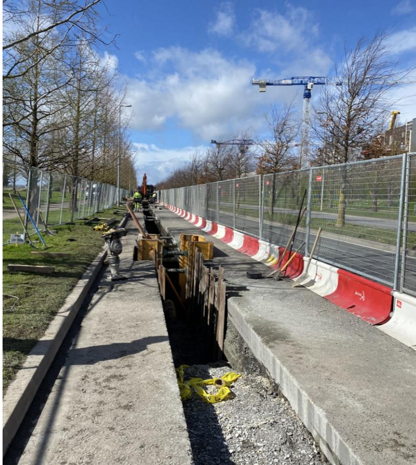
Figure 42: Example of Open Cut Streetworks Excavation for Gas Pipeline
