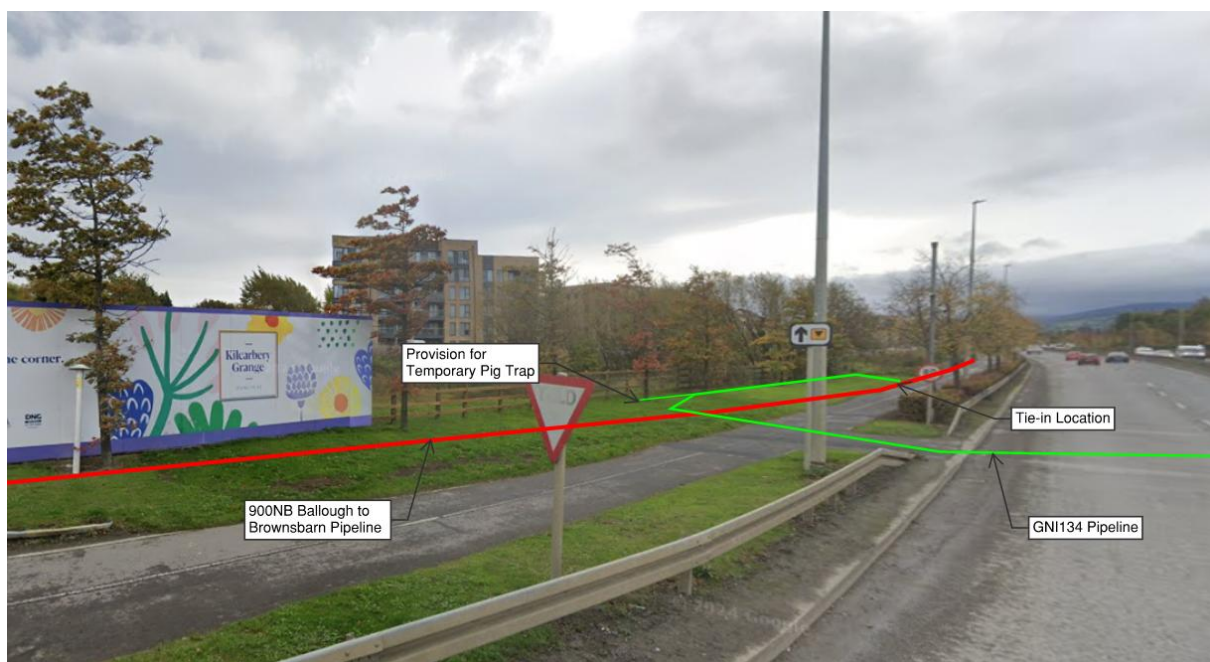
Figure 9 - Tie-in Location Street View
