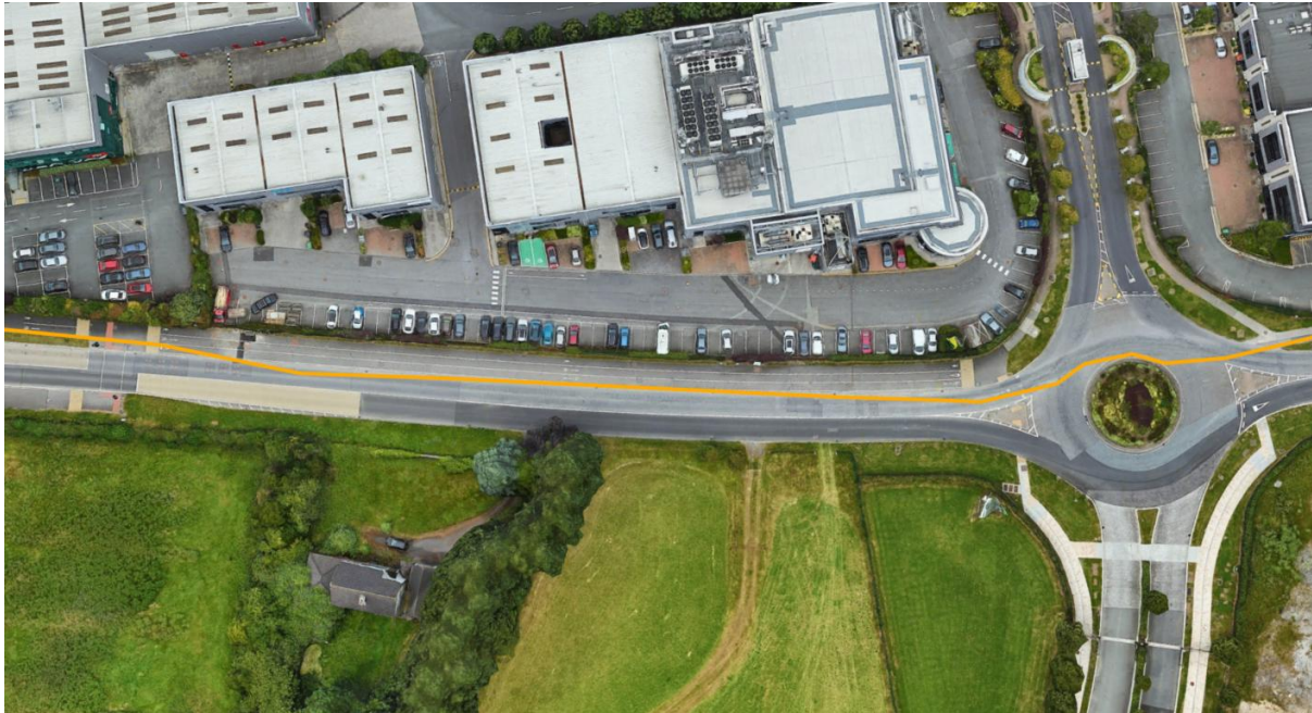
Figure 20 – GNI136 Pipeline re-enters the roadway for a run of 150m after Profile Park roundabout
