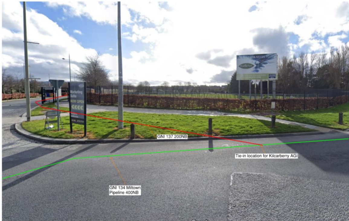
Figure 30 - Tie-in Location Street View
