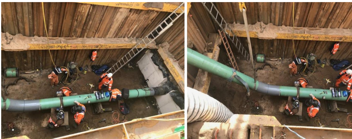
Figure 40 - Example of a Sheet Piled Excavation
