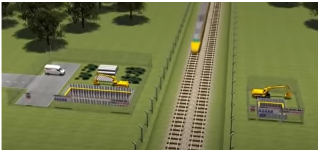
Figure 38 - Typical Auger-boring Set Up for Deep Crossing
