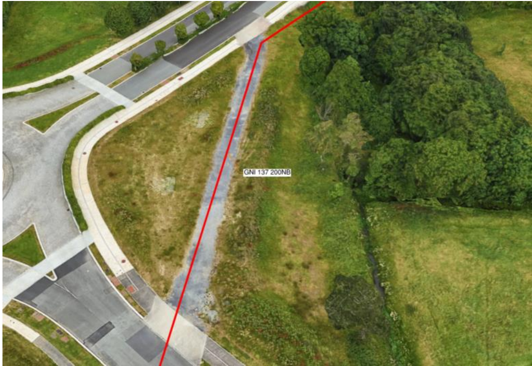
Figure 33 - Pipeline routing through the pathway adjacent to the first roundabout on the Profile Park road
