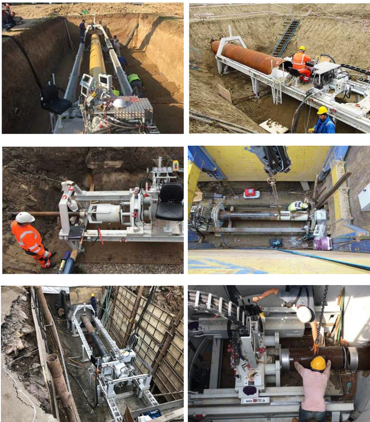
Figure 14: Auger-boring Launch Shaft Construction Setup
