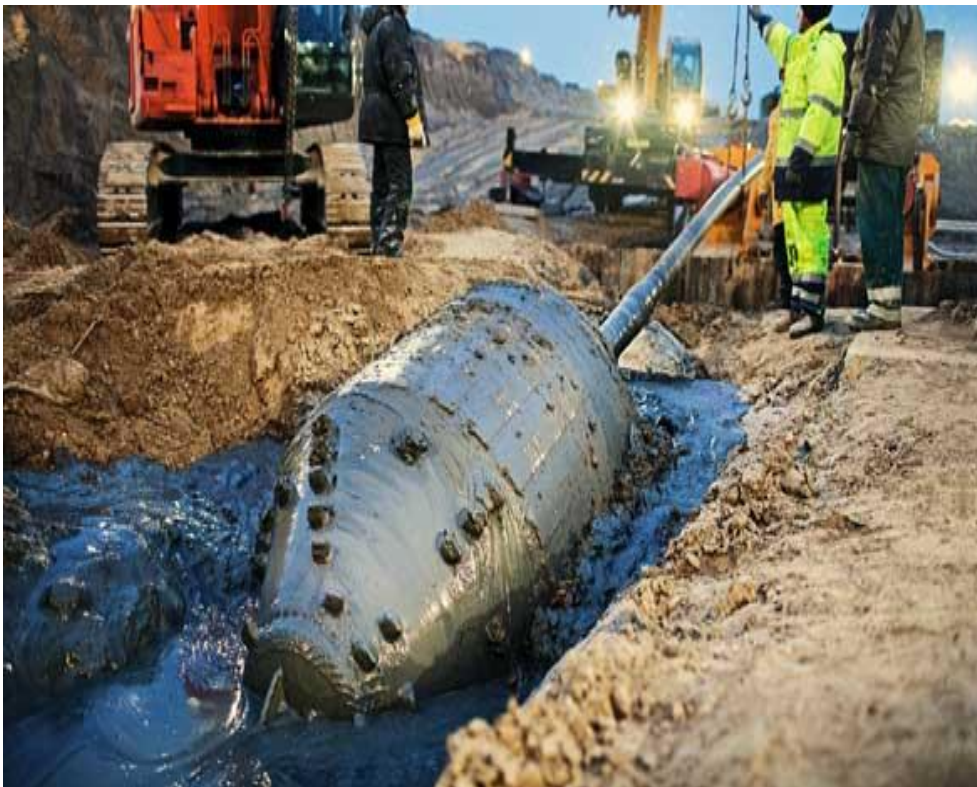
Figure 7: HDD - Hole-opening using a Barrel Type Reamer
