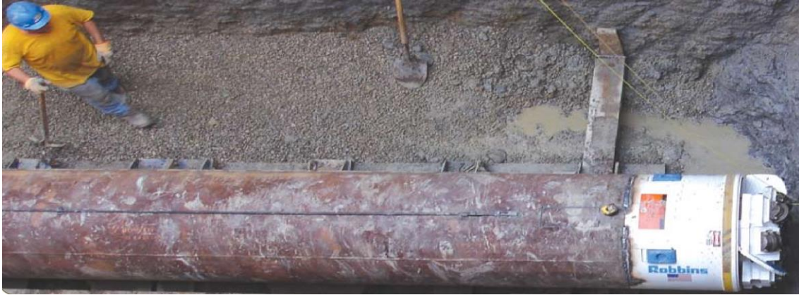
Figure 13: ROBBINS SBU Unit in Use for a Short Hard Rock Crossing
