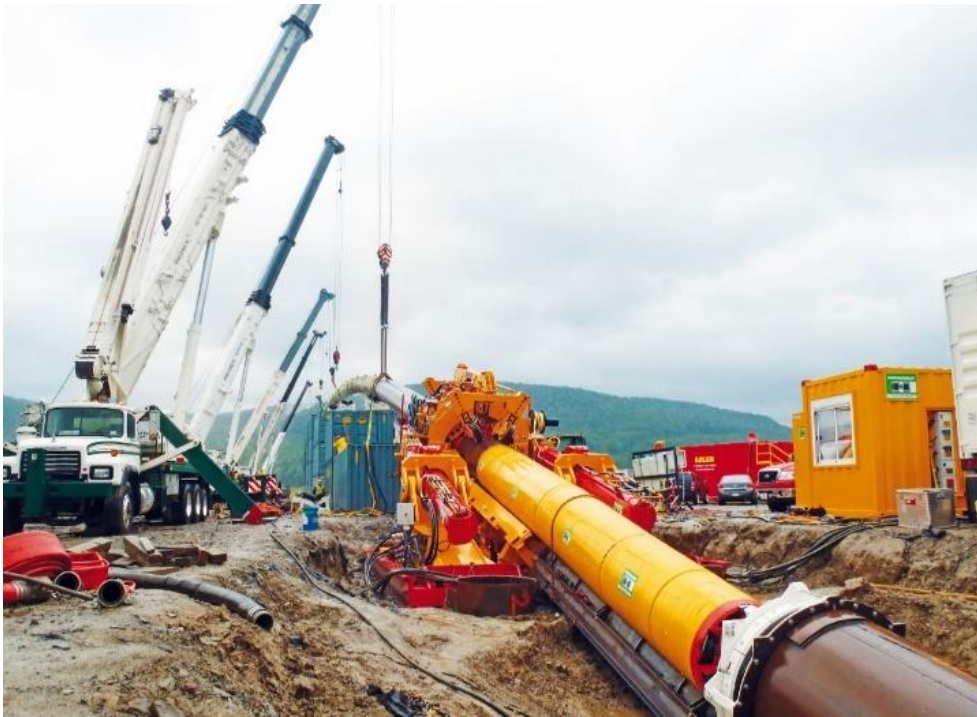
Figure 10: Direct Pipe Micro-tunnelling showing Thruster Rig Installing Pipe-string (entry angle approx. 10°)
