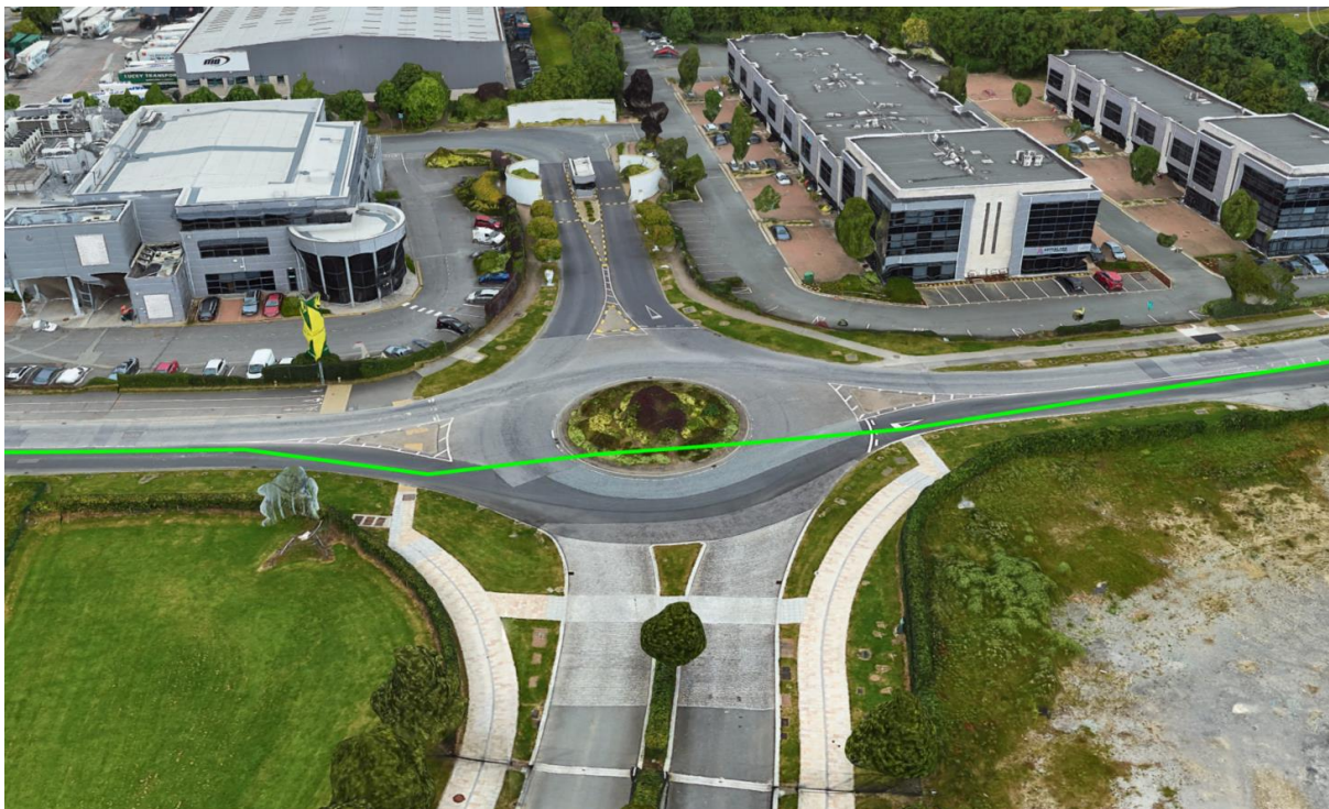
Figure 12 – Profile Park Roundabout
