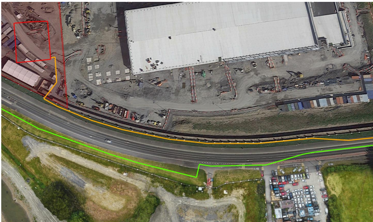
Figure 21 – GNI134 and GNI136 pipelines separate as two high voltage cables enter and run parallel along the R134 roadway
